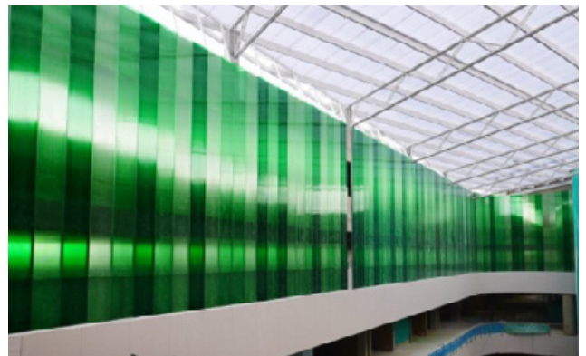
Interior Design - Lighting
