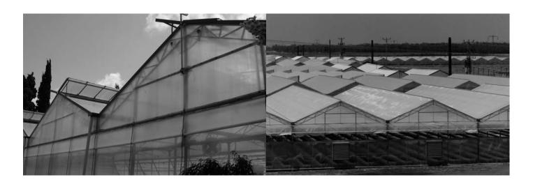
PLASKOLITE Standard 16 mm Ice sheets, combine highly effective thermal insulation with extra strength for low pitch roofing.
